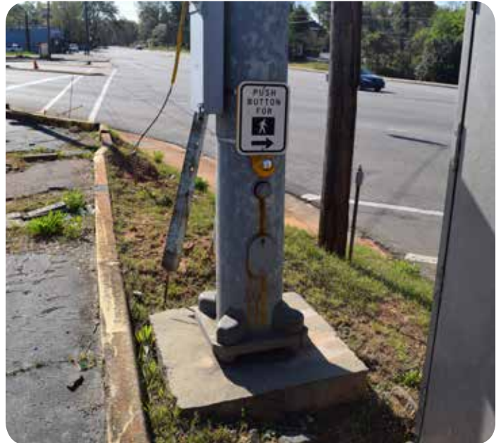
A pedestrian push button placed at the crest of a berm, in front of a utility box, and where sidewalks are lacking prevent pedestrians from being able to use this facility that aids in a safe crossing. This is at the skewed intersection of Clement Drive, River Drive, and Route 16.
