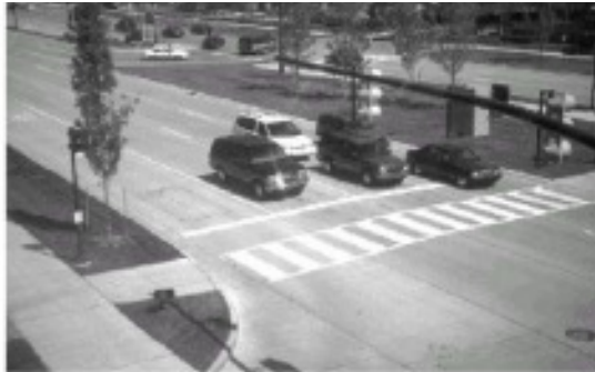
The "ladder" pattern shown above is more visible to motorists and requires less maintenance if painted to allow the tires of motor vehicles
